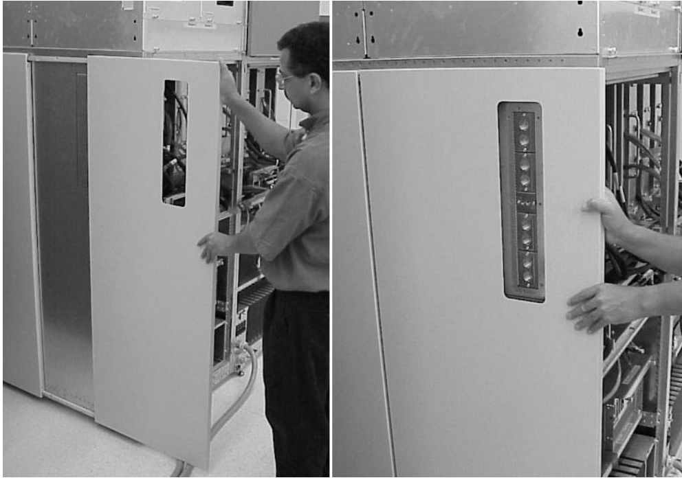
Figure 2-11 Installing New Side Skin
