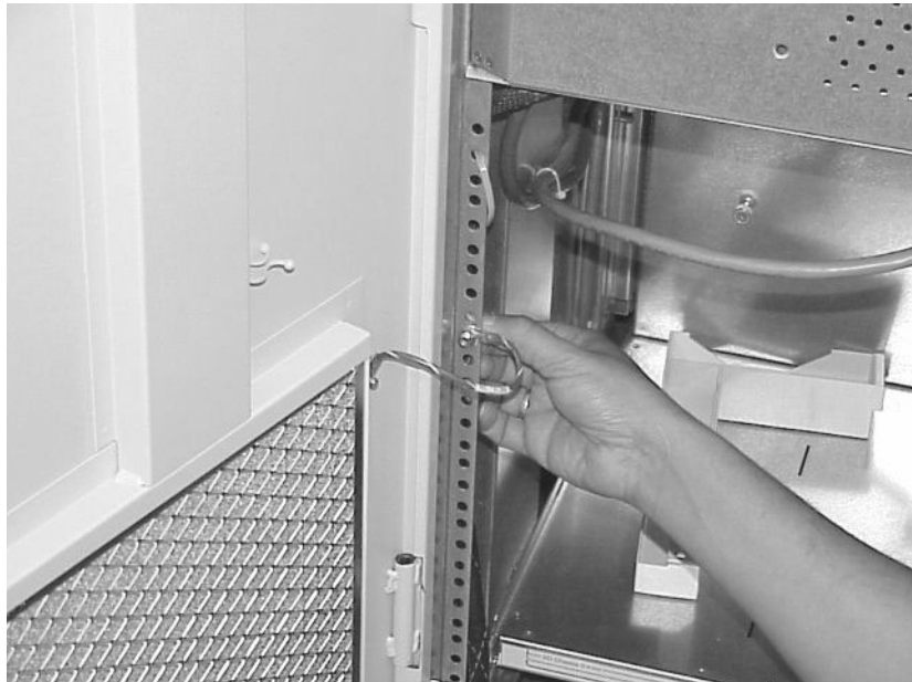
Figure 2-3 Removing Rear Door Grounding Wire
