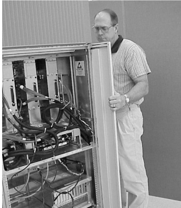
Figure 2-7 Superdome Side Skin Removal
