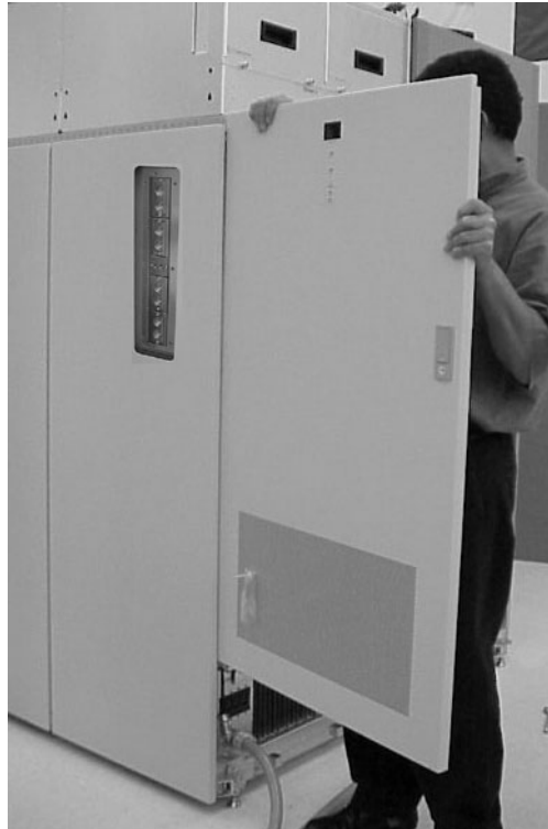
Figure 2-12 Reinstalling the Rear Door
