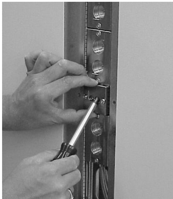
Figure 3-40 Removing the GSP Bus U-PEC
