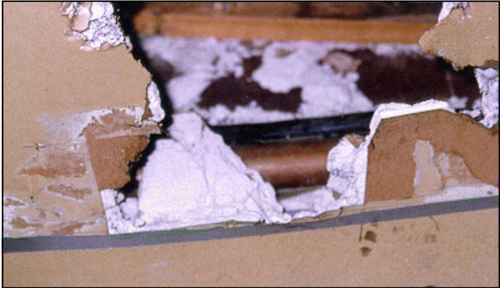
FIGURE 4-2 Subfloor Penetration
