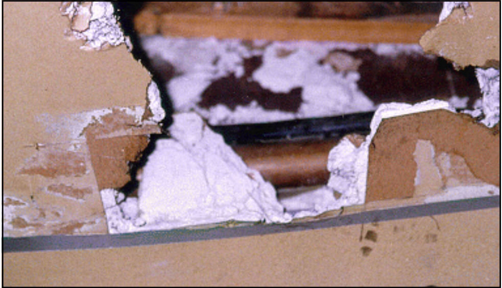
FIGURE 4-2 Subfloor Penetration
