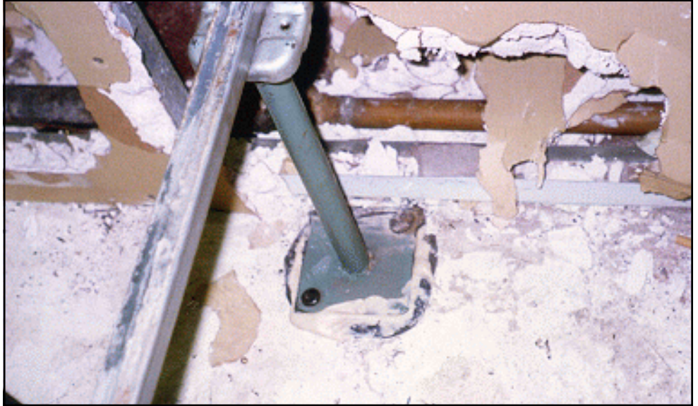
FIGURE 3-6 Subfloor Penetration
