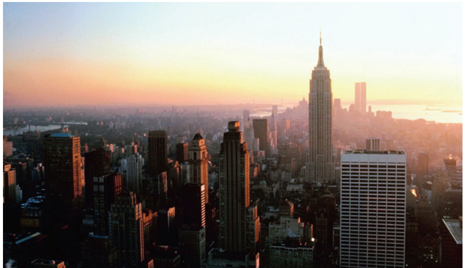
Figure 1. The majority of datacenters support a mixture of high and low-density racks, just as a city skyline features skyscrapers surrounded by hundreds of small and medium-sized buildings.
