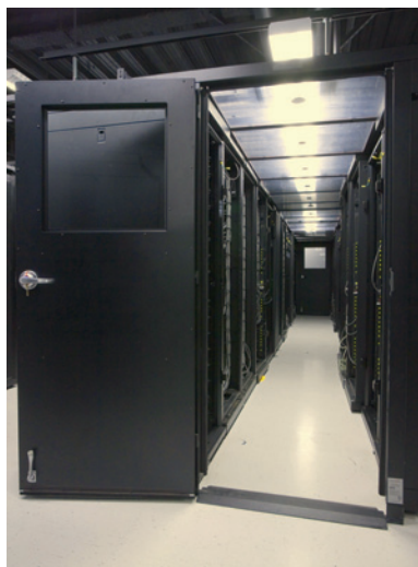
Figure 18. The hot aisle is contained with ceiling tiles and doors at the ends of the pods (left). Two InRow RC units were installed where one was required, providing expansion capacity (right).
