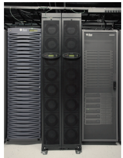
Figure 18. The hot aisle is contained with ceiling tiles and doors at the ends of the pods (left). Two InRow RC units were installed where one was required, providing expansion capacity (right).
